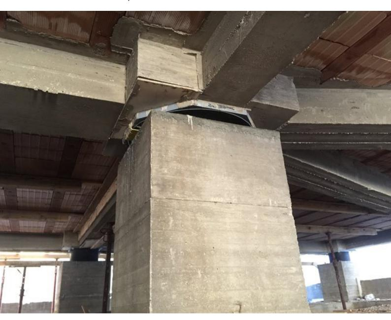
It is easy to see how structural ductility requirements become secondary for buildings designed with seismic isolators at the base.
