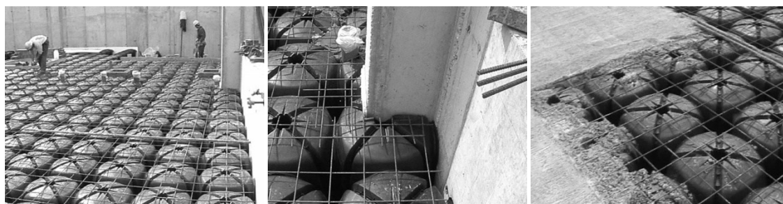
Figure 7 - Assembly stages of the Cupolex floor.
