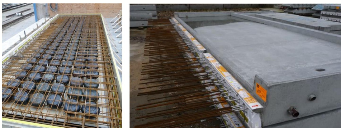
Figure 16 – Precast COBIAx Slabs
